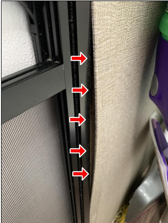
Wall panel rear door in bathroom
