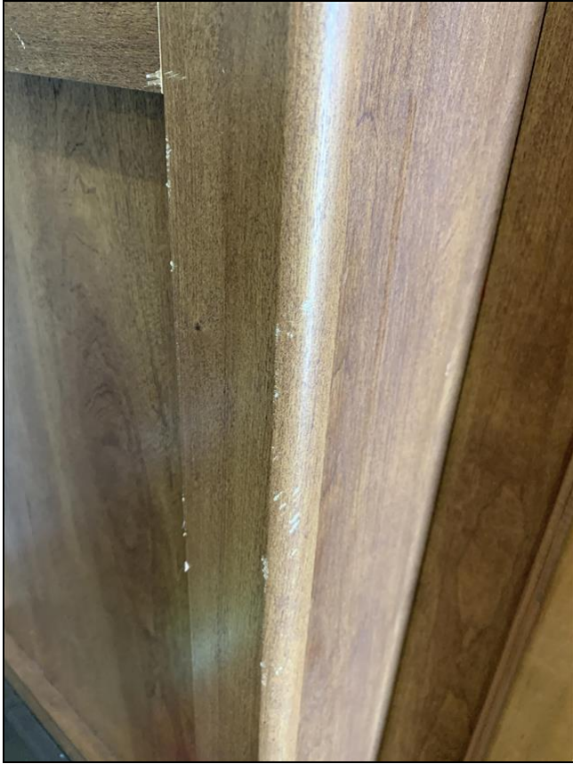
Cabinet on front bedroom wall in main area
