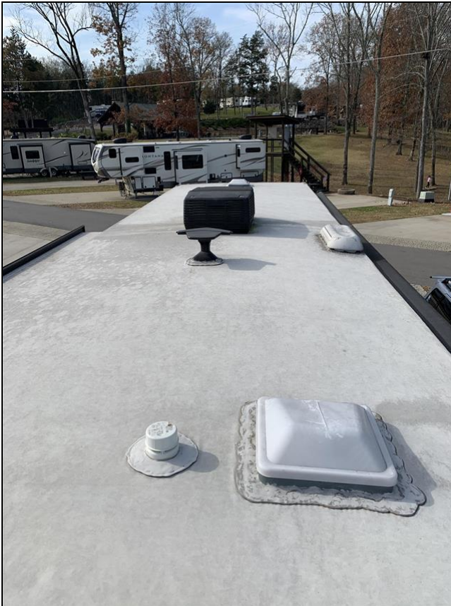
Roof Rear to Front
