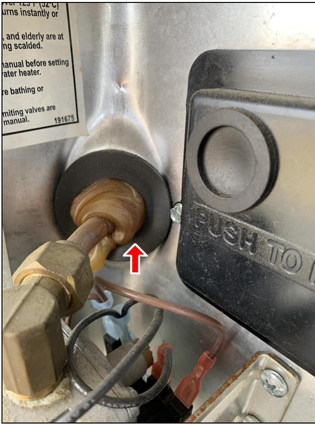
Gas line sealed
